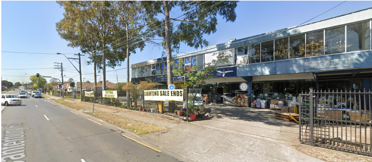
Figure 4 – View of subject building from Canterbury Road c.2023 (note the ample parking available) Source: Google
